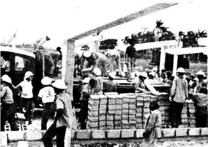
Cubans and Americans working together to build a new school.
