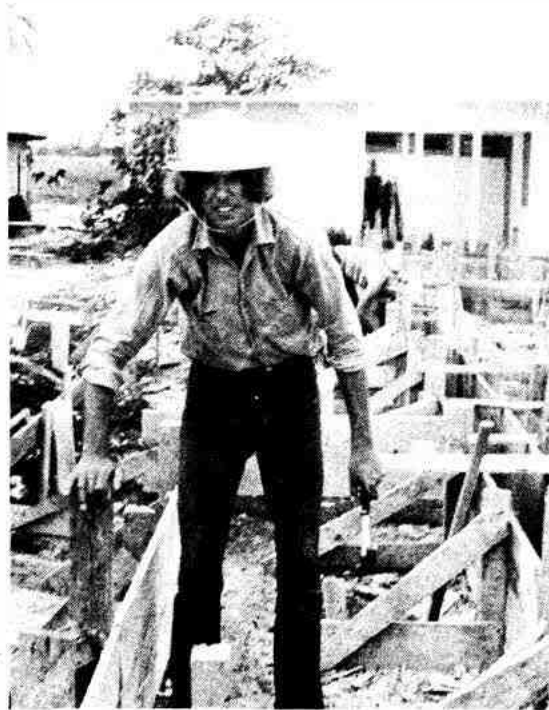
Brigandista building forms for a concrete foundation.
