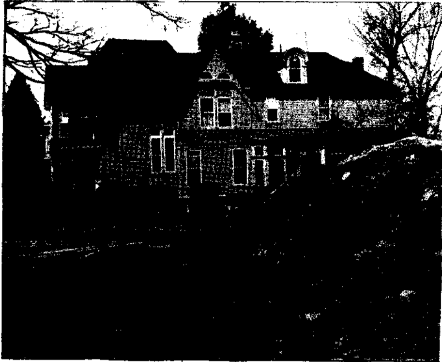
This is how the scene at The Jefferson St. construction site looked before the neighborhood residents got their court injunction.
